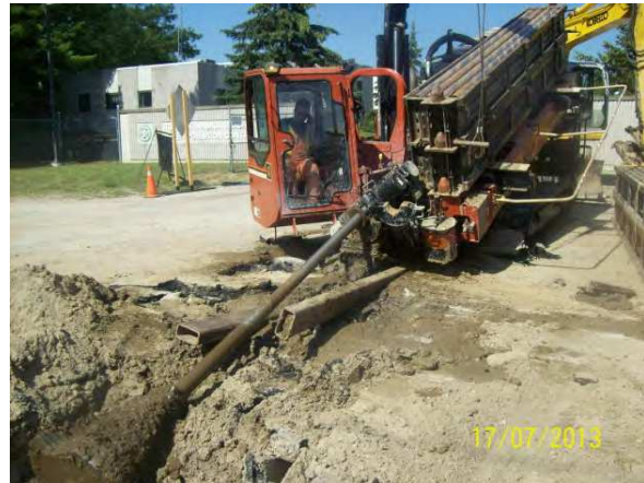
Directional drilling rig
