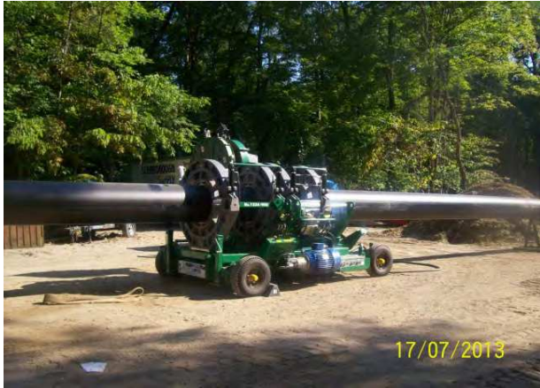
Pipe fusing rig, joining two sections of watermain
