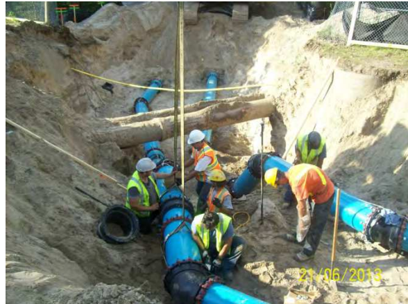
Staff installing flexible pipe
