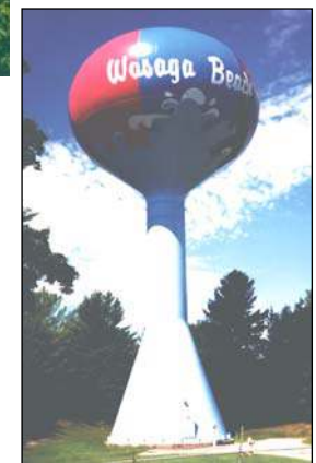
East End Reservoir
