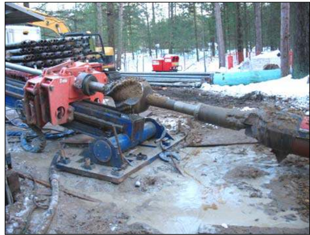
Directional drill equipment.
