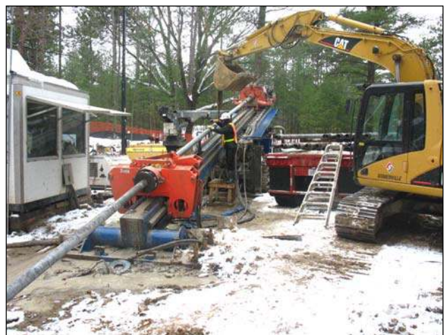
Directional Drilling rig in operation during winter conditions
