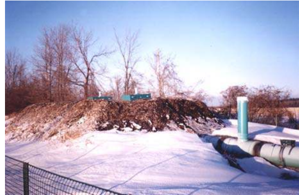
The pilot biofilter bed in the middle of winter
