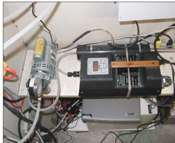
Figure 5 – Rotronic Temperature/Humidity Transmitter (incoming sewer air)
