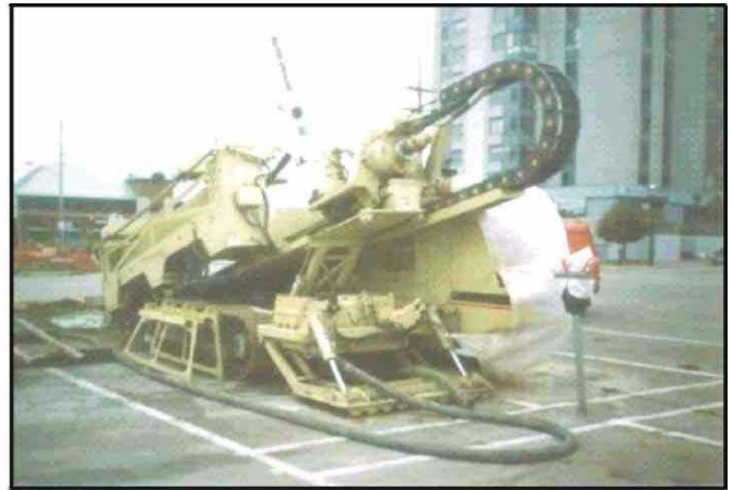
Drilling beneath Bayfield Street.
