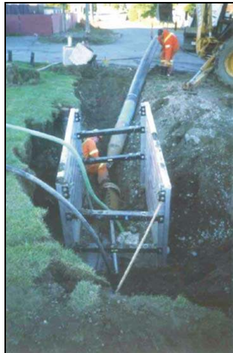
Insertion pit at Toronto Street.
