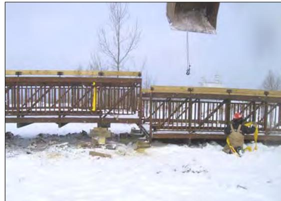
*Splicing the two prefabricated sections.*
