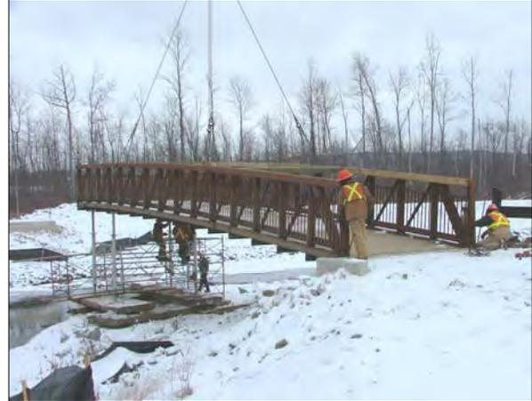
*Aligning the first section with the abutment.*
