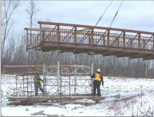
*Lowering the first prefabricated bridge section.*
