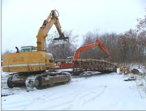
*Moving the prefabricated steel truss bridge.*
