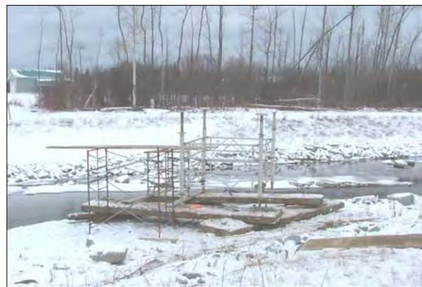
*A temporary scaffold and support structure was erected on the floodway channel bed.*
