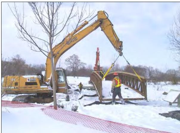
*Positioning the spliced bridge structure.*
