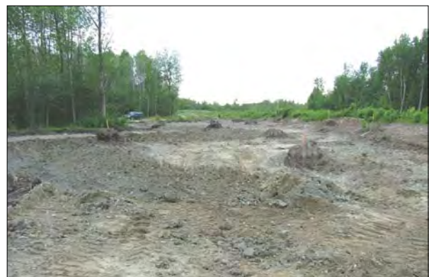
Initial clearing of the work site.
