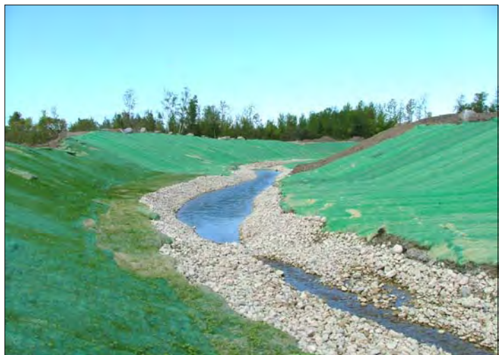
A completed section of Phase III of the Black Ash Creek Flood Control Project showing the seed and erosion control blankets on the side slopes.
