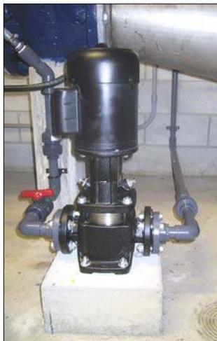
*The chlorine booster pump at the Bayfield reservoir showing the water draw and injector piping.*
