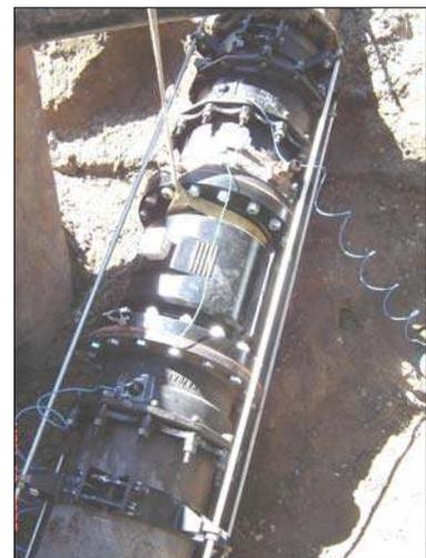
*Electromagnetic flow meter positioned on the common fill/draw line.*
