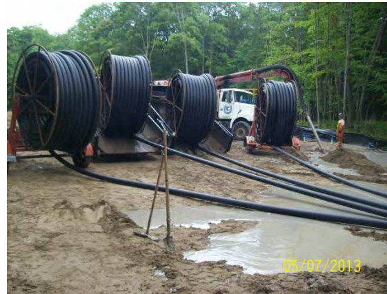
100mm hydro ducts strung underground
