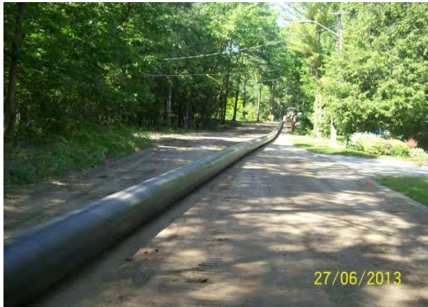
500mm diameter watermain strung along River Road East
