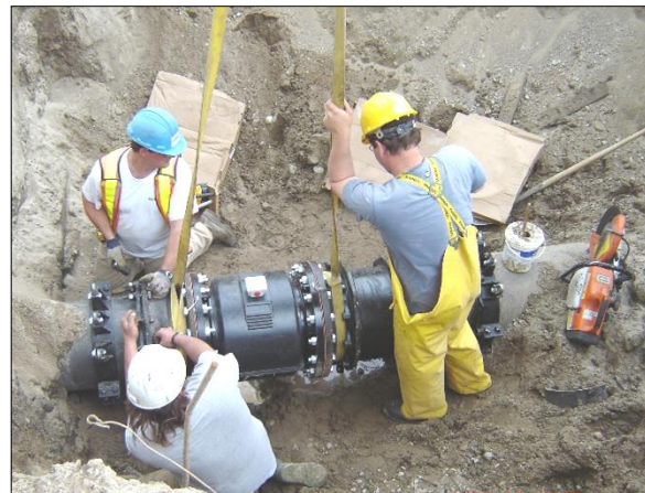
The electromagnetic flow meter being installed on the common fill/draw line.
