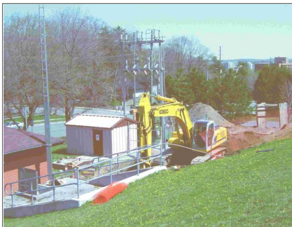
Construction at the Anne Street reservoir.
