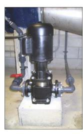
The chlorine booster pump at the Bayfield reservoir showing the water draw and injector piping.
