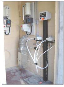
Inside the chlorine room at the Anne Street reservoir showing the chlorinators, weigh scales, vent and gas sensors.
