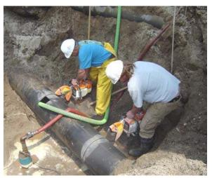
Construction personnel cutting a section of the common fill/draw line to provide a space for the flow meter at the Mapleview Elevated Tank.
