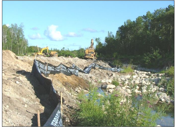
The existing creek bed (at the right) was protected while construction of the new alignment continued.
