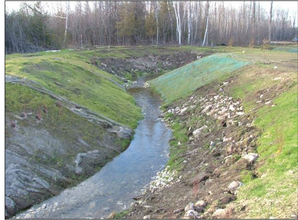
A completed section of the new Petun branch meandering stream bed, which parallels the main channel for 500 metres
