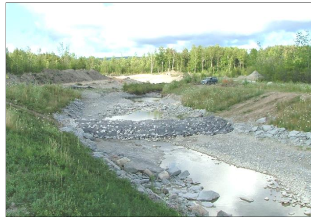
A silt cofferdam was constructed at the upstream limit of Phase II to prevent sediment migration.
