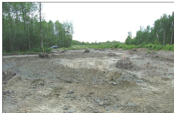
Initial clearing of the work site.
