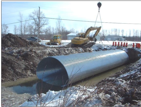
Positioning the multi-plate steel culvert extension.
