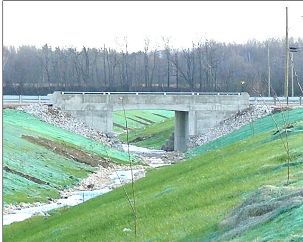
The completed Sixth Street Bridge
