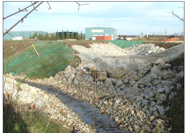
This photo shows one of the rock revetments, completed slopes and landscaping.
