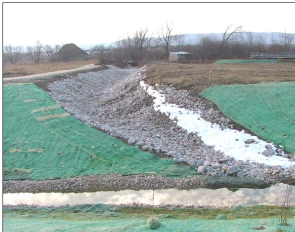
A weir was constructed at the original merging point of the Petun to divert flow into the new stream bed.
