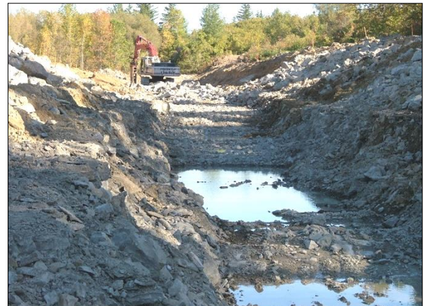
Rock excavation for the new channel alignment.
