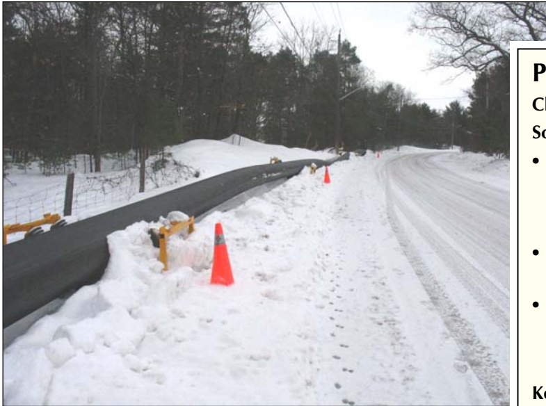
Fused watermain ready for installation by directional drilling.
