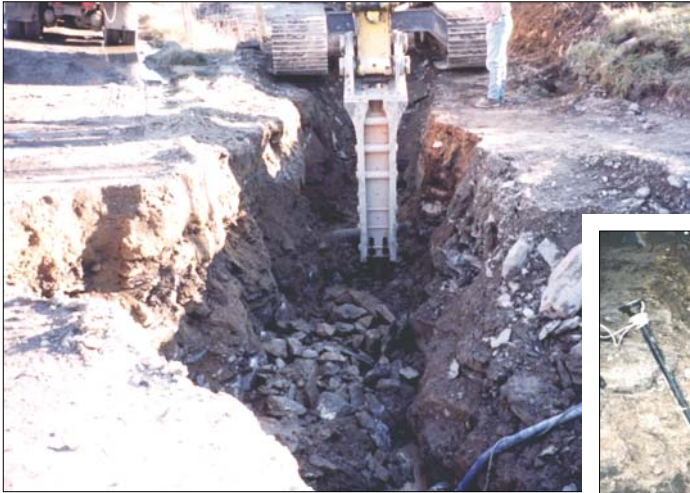
Extensive rock excavation was required along the entire corridor.
