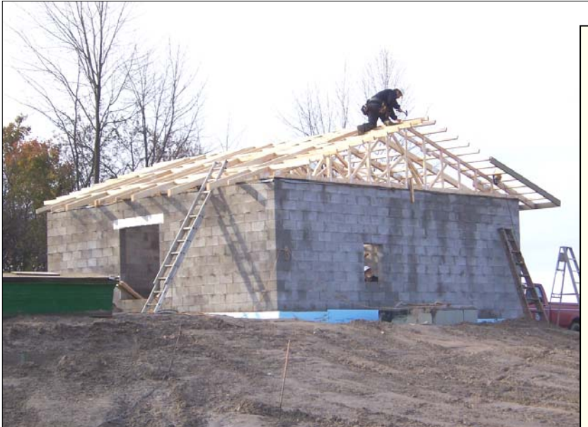
Control Building under construction
