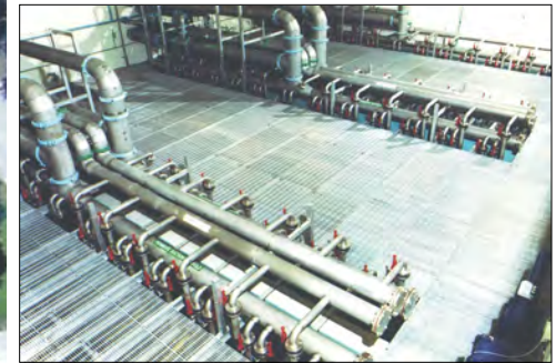
Raw water basins containing filtration cassettes.
