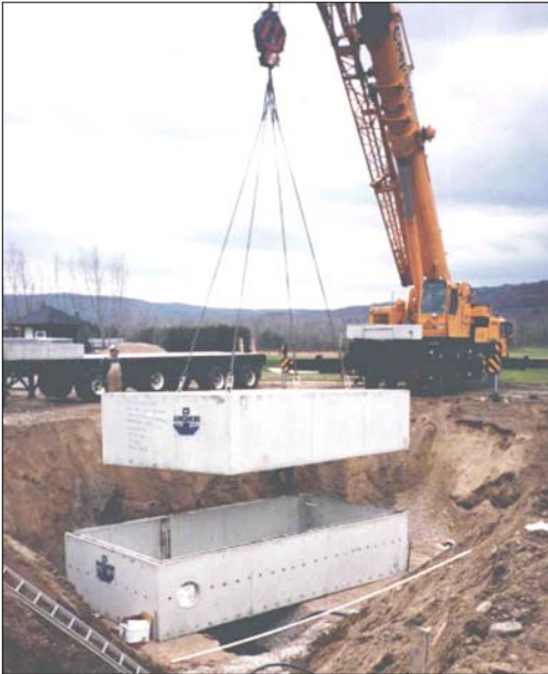
Placement of booster station precast concrete sections
