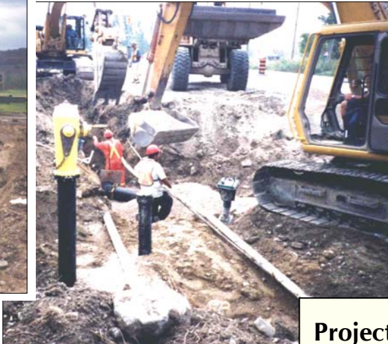
Installation of the 300-mm watermain along Osler Bluff Road
