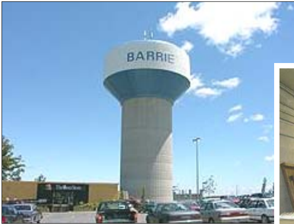
Maplevue elevated reservoir.
