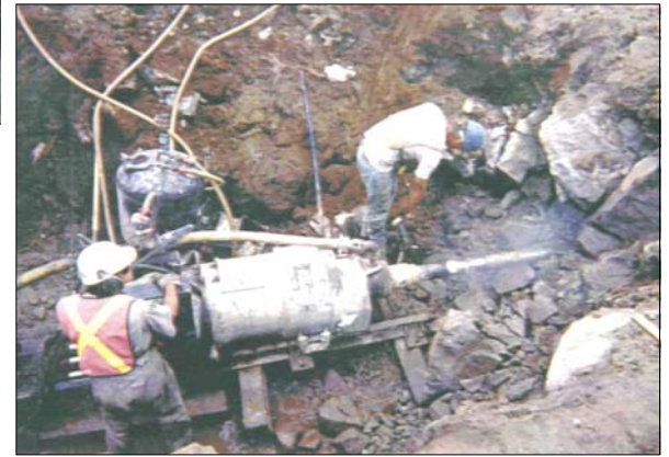
Preparing a water service borehole using a horizontal rock-drilling rig.
