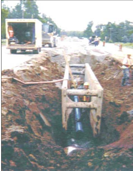
Traditional trench open-cut method for laying water main pipe in Elizabethtown.
