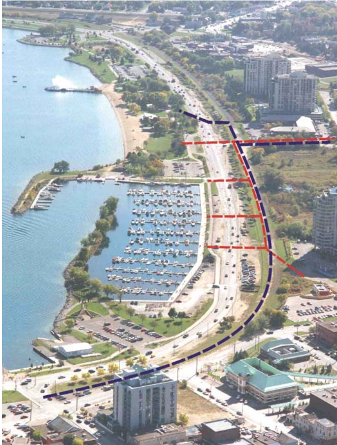
Barrie's waterfront showing the location of the transmission main (purple dashed line) and the distribution main (red dashed line).
