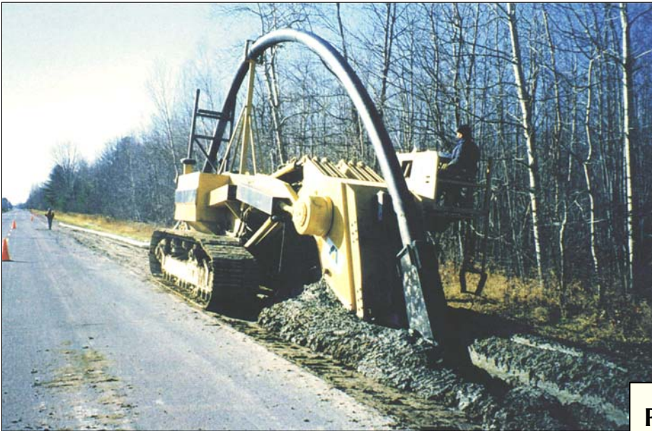
Chain trencher installing HDPE pip
