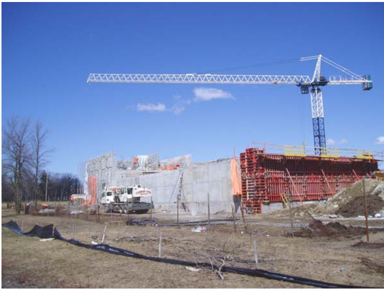
Spring of 2008 - WPCP under construction
