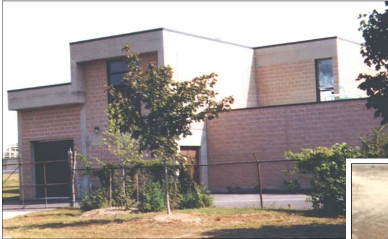
New headworks building housing the new aeration blowers and control room
