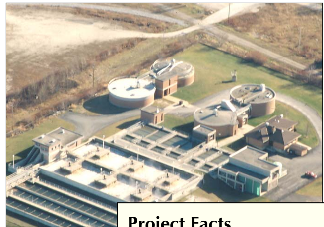
Collingwood Water Pollution Control Plant
