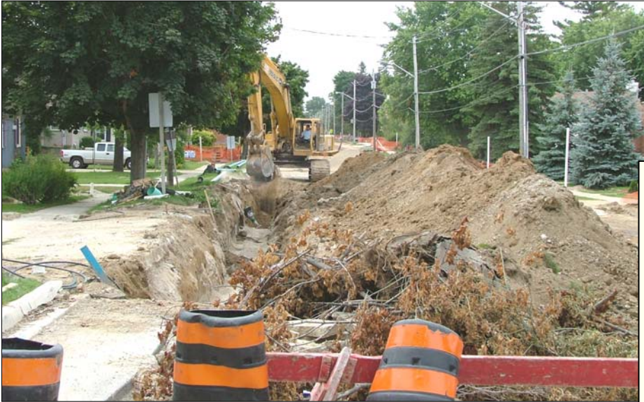
Reconstruction of Bruce Street in Thornbury.
