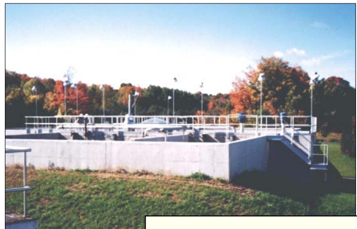
Stage I and II Digester Building
