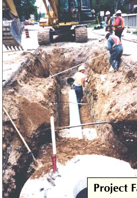
Installation of new sanitary sewer
