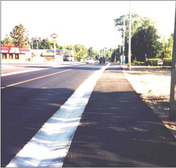
Completed full-width road reinstatement
