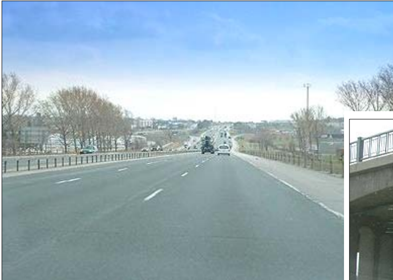
Highway 400 runs through the centre of Barrie.
