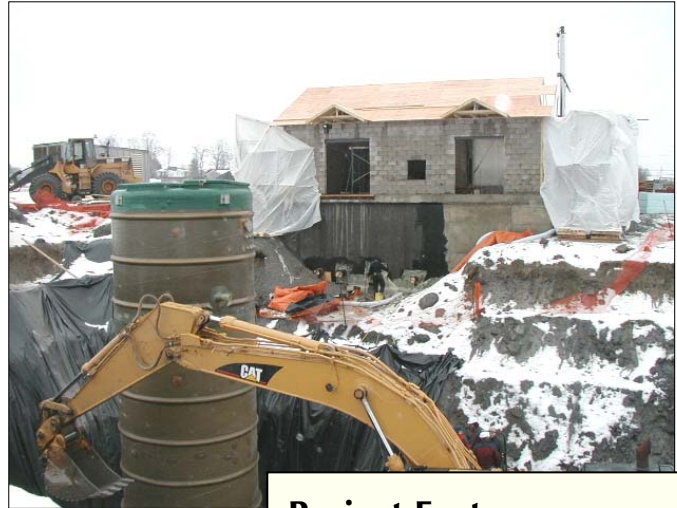
The photo above shows the completed pump station. Construction of the pump house building, piping and the wet well are shown in the photo at the right.
