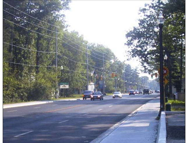
Looking East on Mosley Street showing the new four-lane urban cross section, curbs and sidewalks, street lighting and the new traffic lights at 32nd Street.
