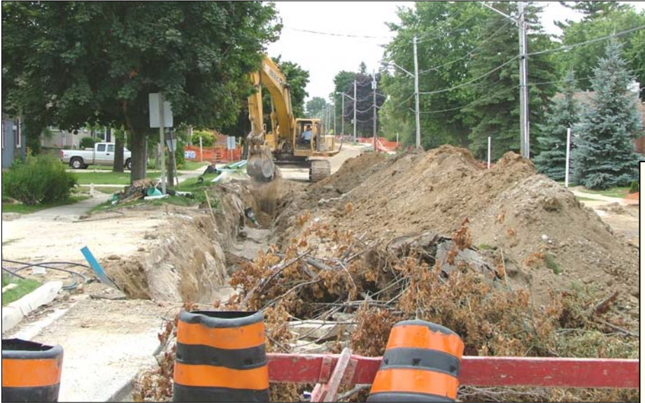
Reconstruction of Bruce Street in Thornbury.
