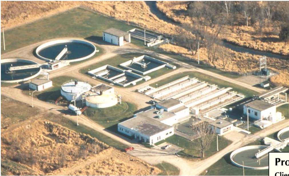
City of Orillia's Wastewater Treatment Centre – designed by the Ainley Group
