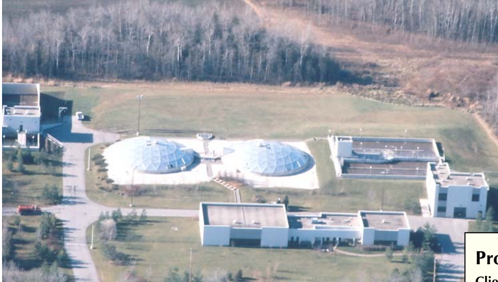
Innisfil's Water Pollution Treatment Plant
