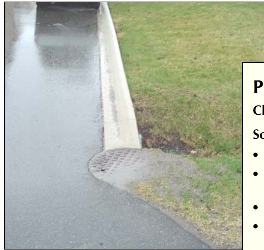
Maintenance holes located in roadside ditches and gutters were the major source of surface water inflow into the sewer-shed.
