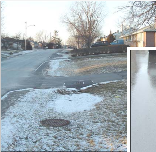
Maintenance holes located in roadside ditches and gutters were the major source of surface water inflow into the sewer-shed.
