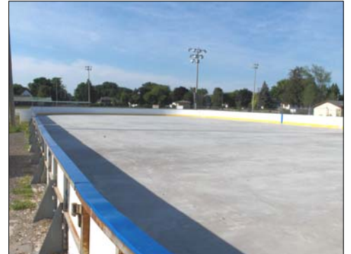
Refurbished 200 ft x 85 ft. outdoor ice pad.
