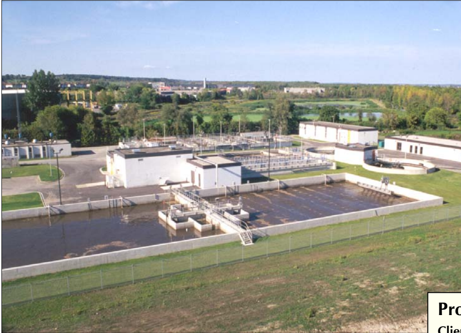
Bradford West Gwillimbury Sewage Treatment Plant
