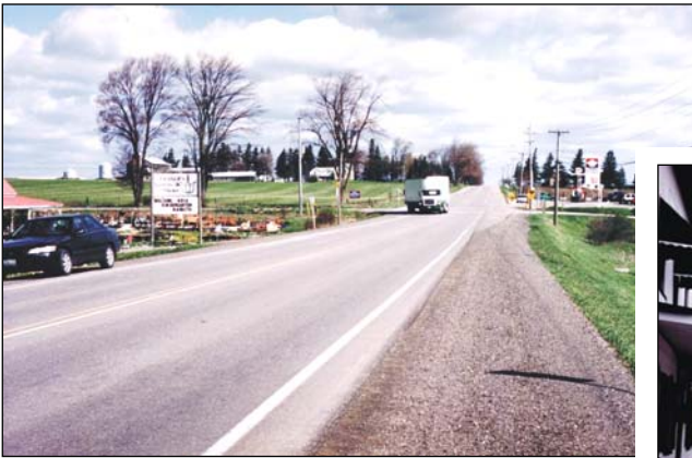
Intersection of Country Road 27 and County Road 1 – a left-turn lane was needed to improve operations and reduce the potential for collisions.
