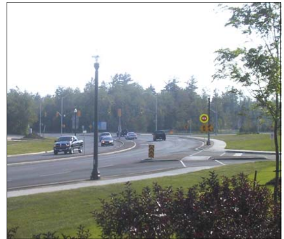
Looking east along Mosley Street towards the new signal lights installed at Puccini Drive. The photo also shows the new street lights, sidewalks, curb and gutter and landscaping.
