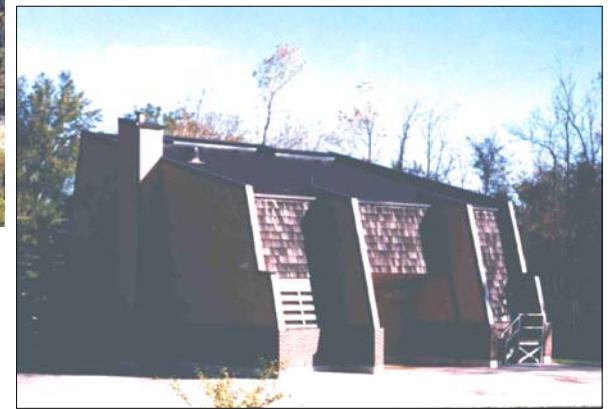
Existing Craigleith Pumping Station
