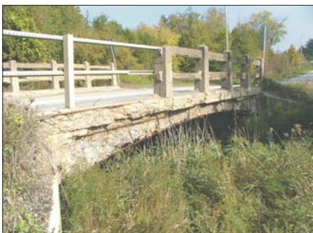
Bailey Creek Bridge
