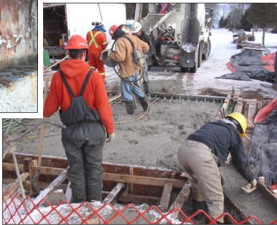
Pouring the deck – December 30, 2005.
