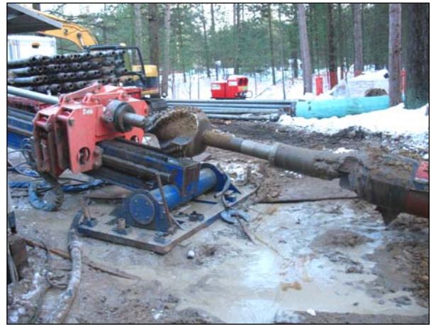
Directional drill equipment.
