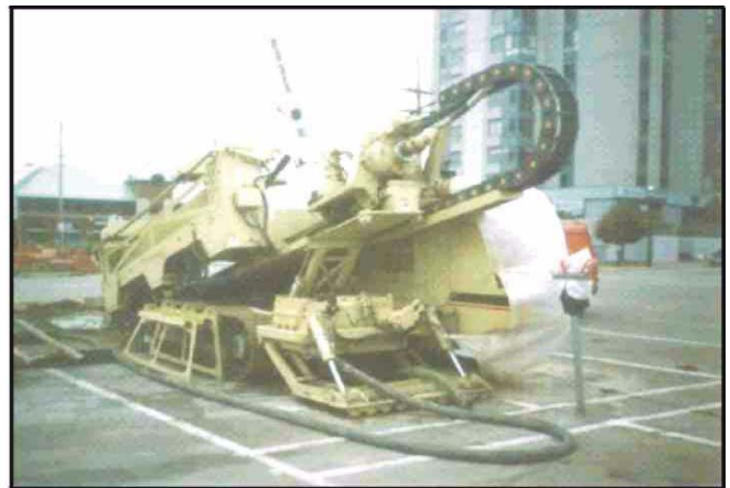
Drilling beneath Bayfield Street.
