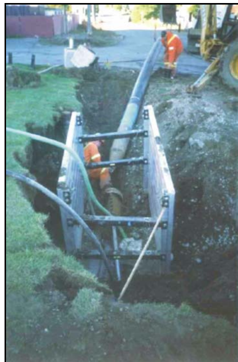
Insertion pit at Toronto Street.
