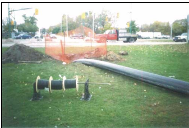
Hydrant lead beneath Lakeshore Drive.
