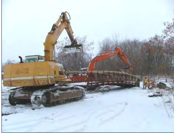
Moving the prefabricated steel truss bridge.
