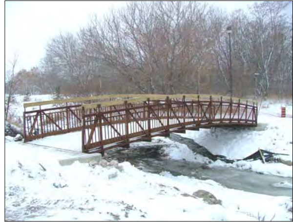
Site No. 2 completed installation.
