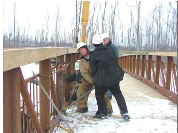
Splicing the sections together.
