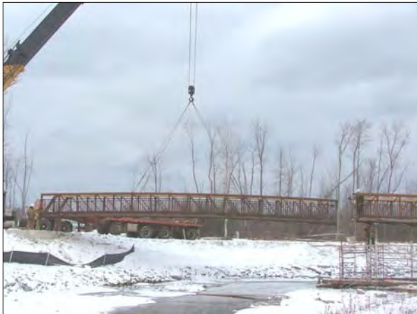
Lowering the second section of bridge.
