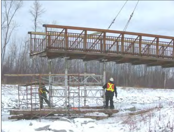
Lowering the first prefabricated bridge section.
