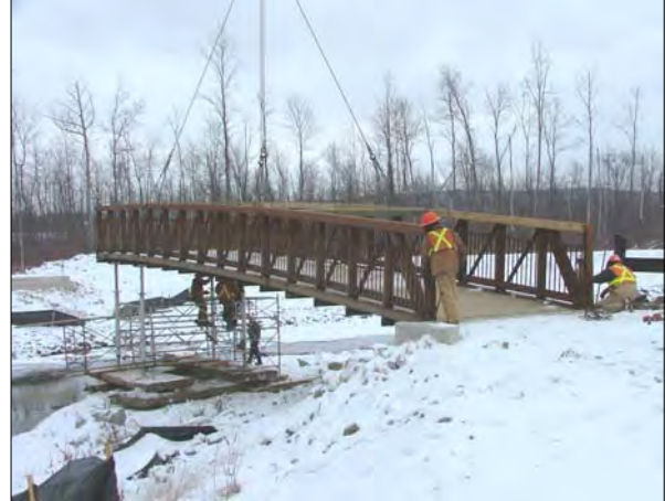
Aligning the first section with the abutment.
