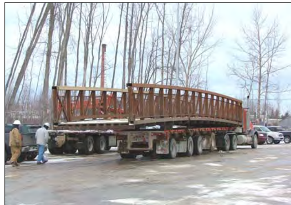
A section of prefabricated bridge arriving on site.
