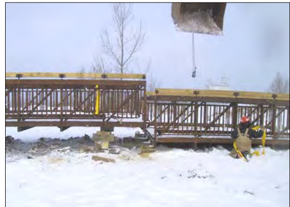
Splicing the two prefabricated sections.
