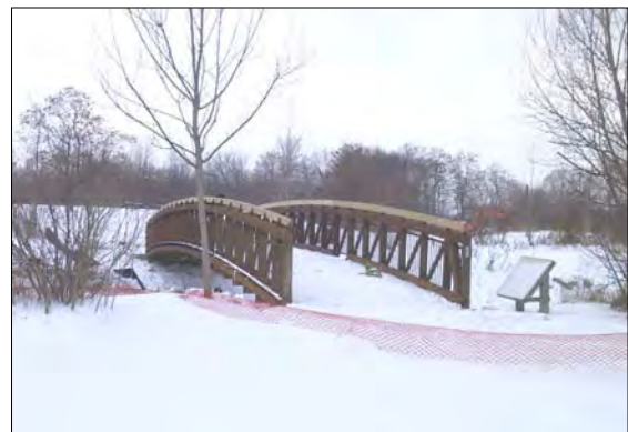
Site No. 1 completed installation.
