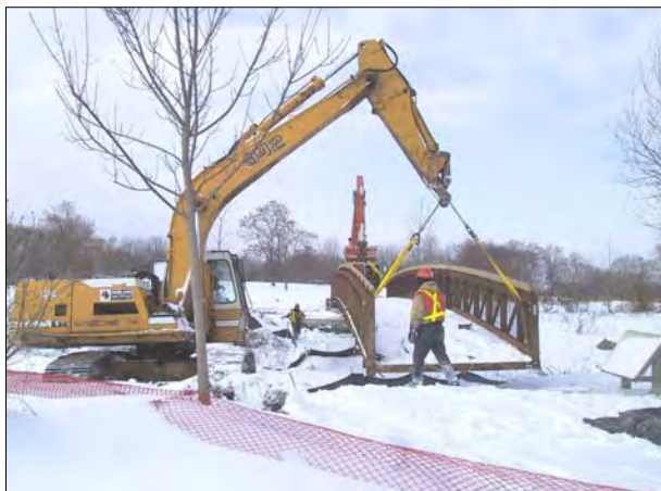
Positioning the spliced bridge structure.
