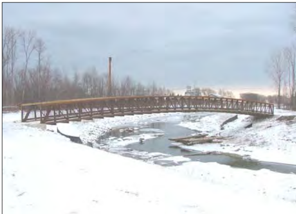
Site No. 3 completed installation.
