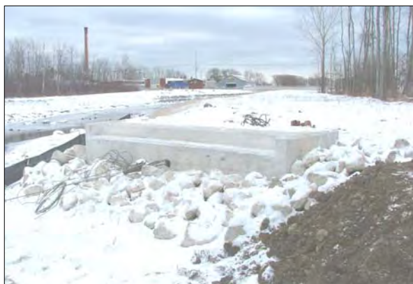
One of the concrete abutments.
