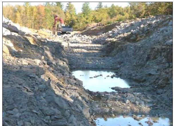
Rock excavation for the new channel alignment.
