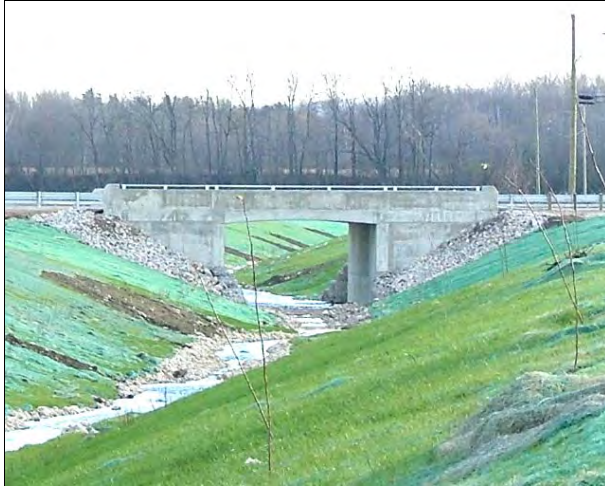
The completed Sixth Street Bridge
