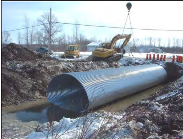
Positioning the multi-plate steel culvert extension.
