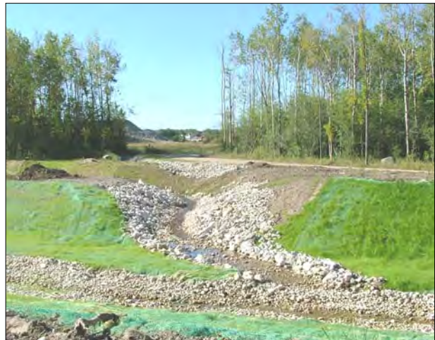
The Petun branch outletting into the main channel
