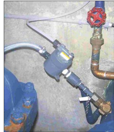
The injector and injection point installation at the Anne Street reservoir.
