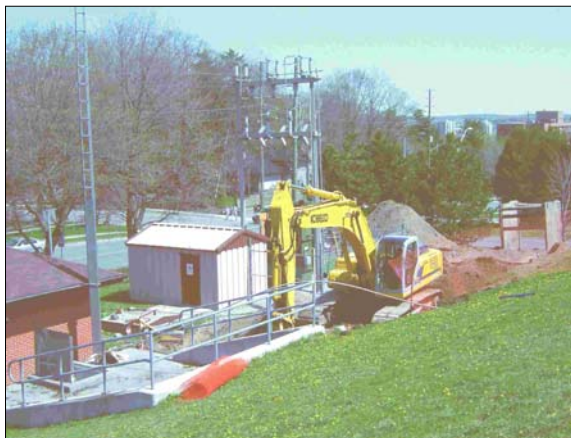
Construction at the Anne Street reservoir.
