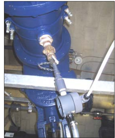
The injector and injection point installation at the Mapleview reservoir.
