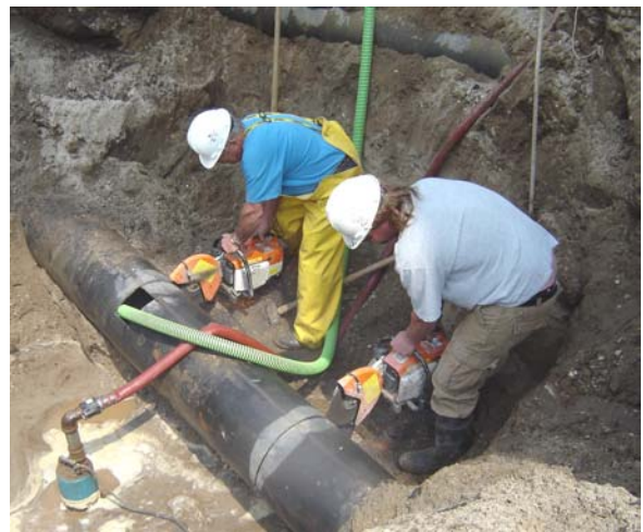
Construction personnel cutting a section of the common fill/draw line to provide a space for the flow meter at the Mapleview Elevated Tank.
